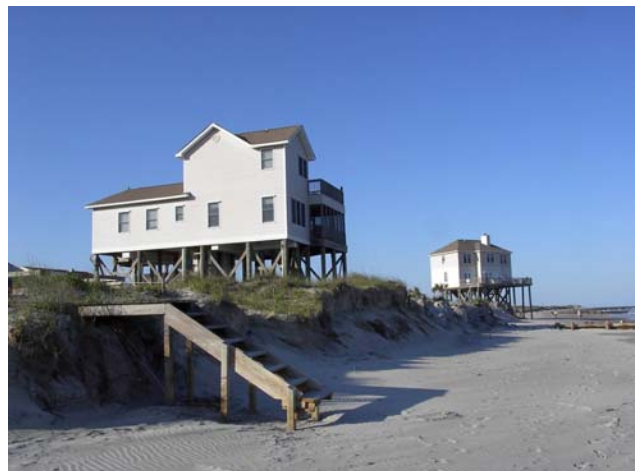
Photos 33 to 35. Most states show flexibility on removal of buildings on the beach as a result of erosion. Top: Westerly, Rhode Island (March 2003). Middle: Kitty Hawk, North Carolina (June 2002). Bottom: Folly Beach, South Carolina (April 2004). Photo source: ©James G. Titus, used by permission.
