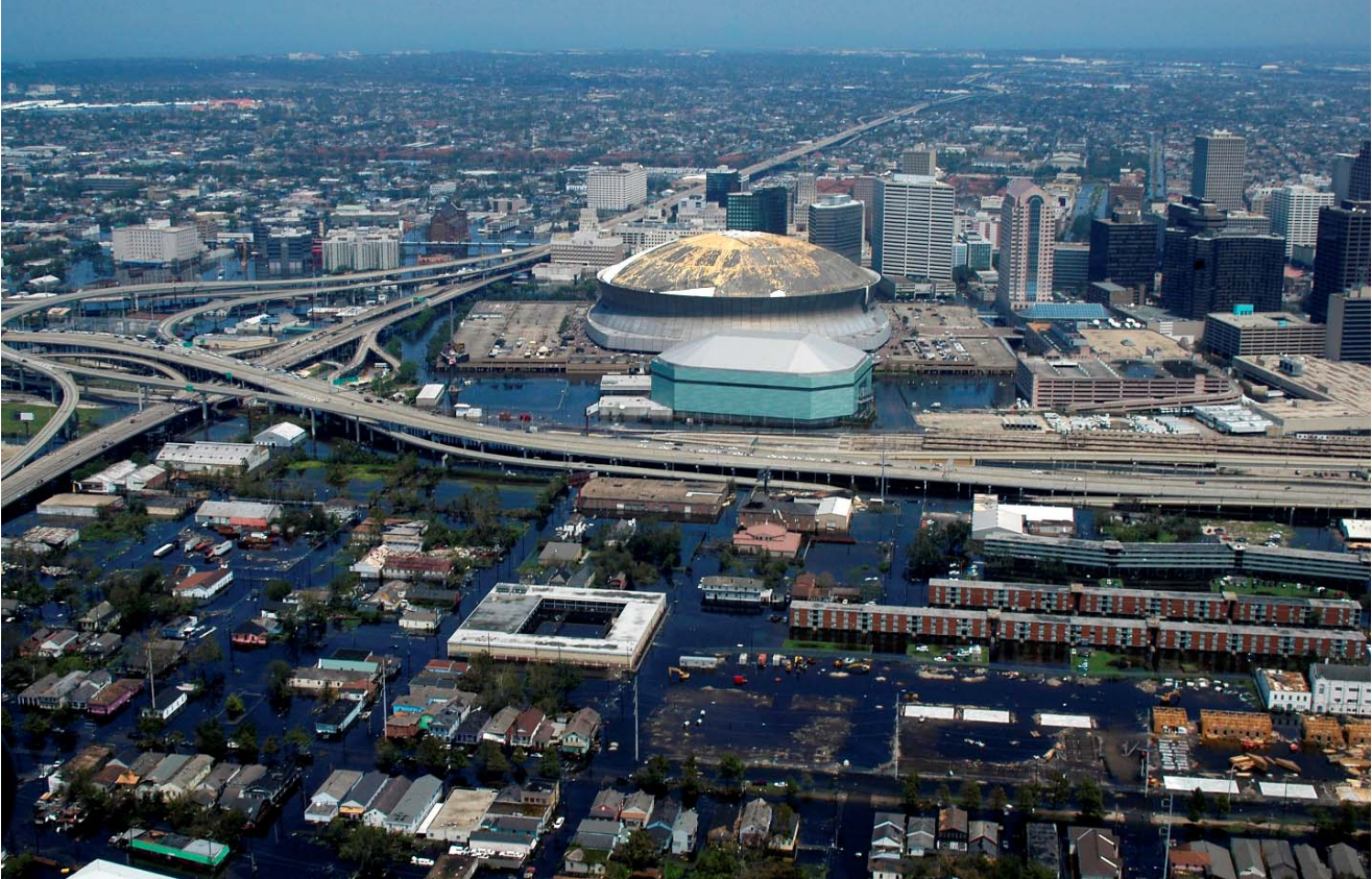
Photo 29. Living Below Sea Level Can Be Hazardous if Shore Protection Fails. Downtown New Orleans after the failure of dikes along the Industrial Canal. (Aerial view from a U.S. Navy helicopter. August 31, 2005.)
