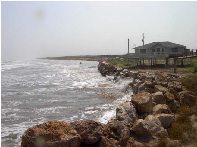
Photos 16 to 18. Shoreline armoring can make vehicular and pedestrian access along the shore impractical. Top left: a seawall protecting some high-rise buildings along the Gulf of Mexico on North Padre Island prevents automobile traffic on the beach (March 2010). Top right: At first, traffic was restricted to one-way (March 1998). Bottom: a stone revetment makes walking along the shore impractical north of Surfside, Texas (May 2003). Photo source: ©James G. Titus, used by permission.
