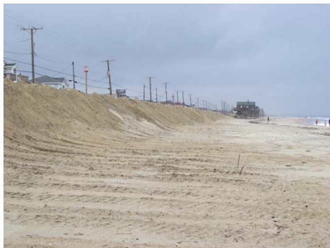
Photos 6 to 8. Retreat. Houses along the shore in Kitty Hawk, North Carolina, where regulations prohibit seawalls. Geotextile sand bags protect a septic tank buried in the dunes. Homes stand on the beach until the septic system fails. Top: June 2002. Middle: October 2002. Bottom: June 2003. Photo source: ©James G. Titus, used by permission.
