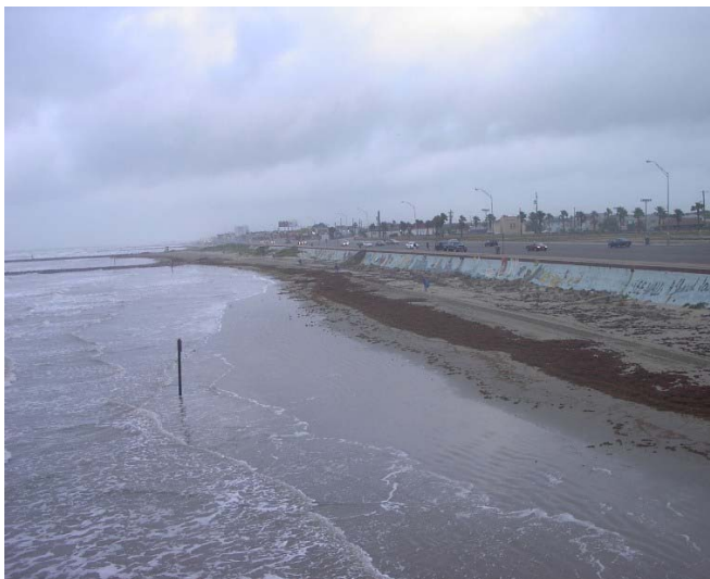
Photo 5. Galveston Seawall. (May 2003). Photo source: ©James G. Titus, used by permission.
